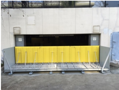
New floodbreak at 6386 Alvarado Court
