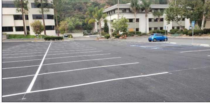
Renovated Parking Lot at Alvarado Research and Professional Center
