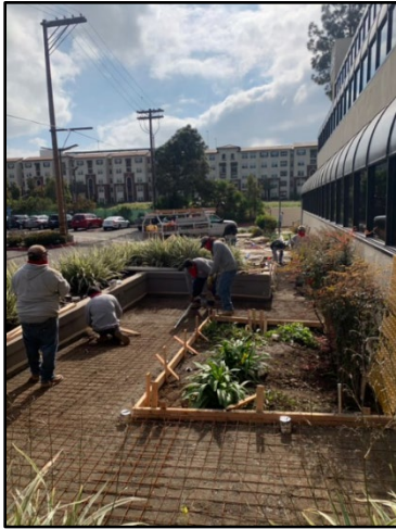
6386 Alvarado Court (Exterior ADA ramp) – During Construction
