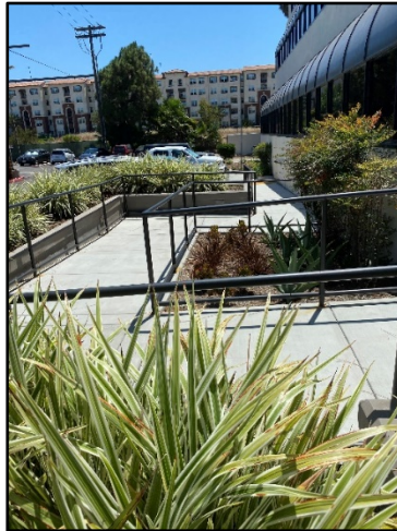
6386 Alvarado Court (Exterior ADA ramp) – After
