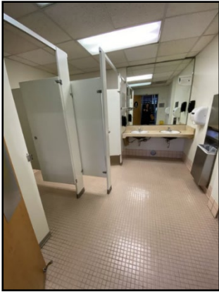
6505 Alvarado Road (Restrooms) – After: Includes new LED lighting, low flow toilets, baby changing tables in both restrooms and sensor faucets.
